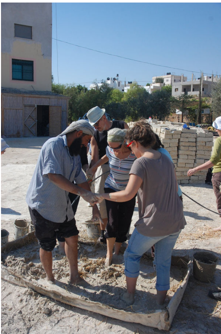
Mixing cement for bricks at Auja Eco-Centre
